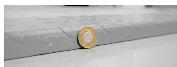
Threshold not exceeding height 25 mm!
